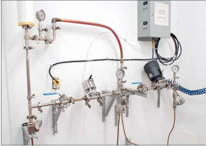
Steam cycle testing of Diaphragms
